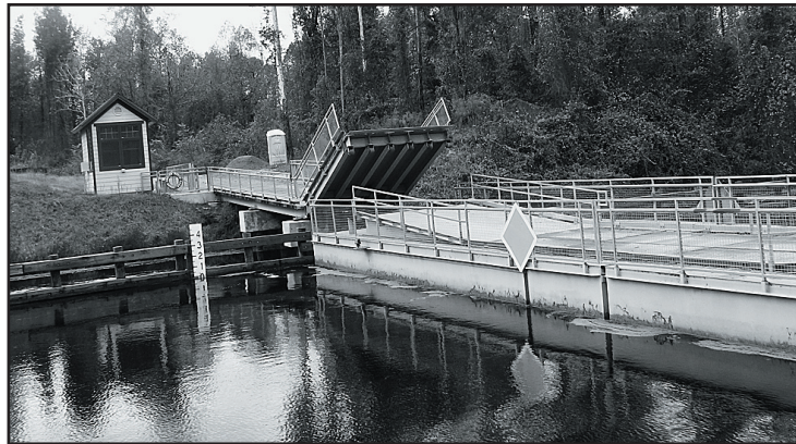
The bridge access to Dismal Swamp Photo: Bob Sowa
